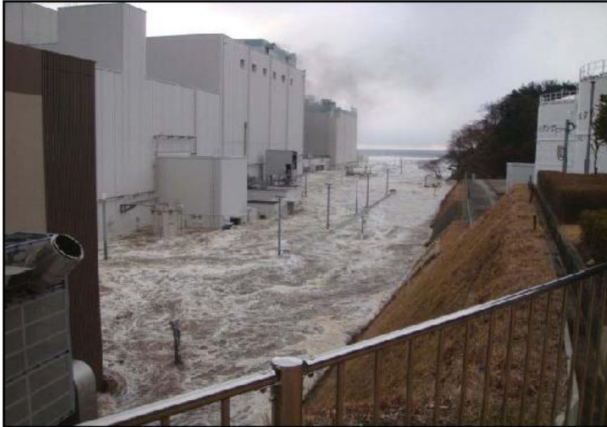
2 to 3 m inundation height on the side of unit 1 building.
