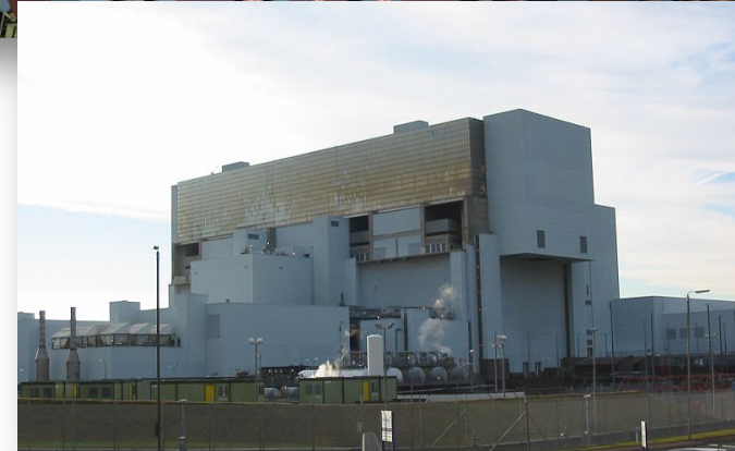
Torness (Scotland UK) (1988) (Built only in the UK)
